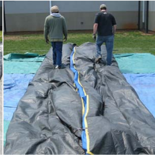
Step 4: After folding the Inflatable twice lengthwise, walk out air towards Ports (Blower tubes).
